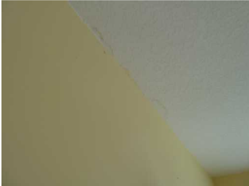
Ceiling in Right Front Bedroom
