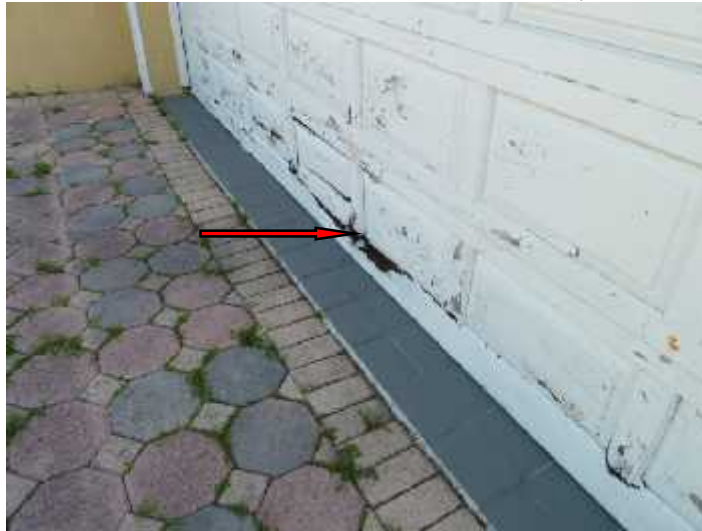
Photo: View of the Exterior of the Garage Door
