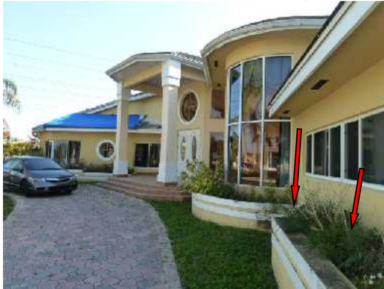
Photos: View of the planters at the front elevation.
