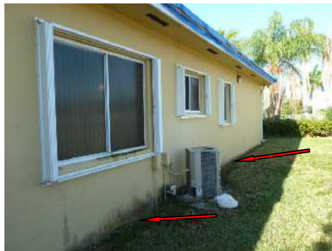
Photo: View of the North Elevation.
