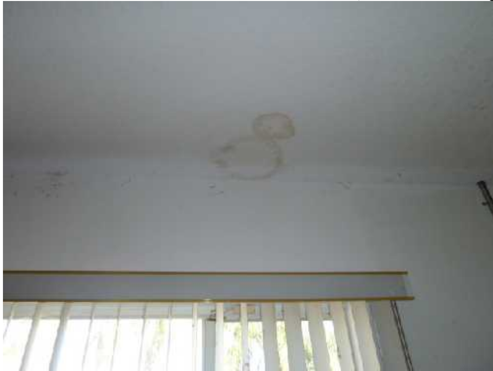
Ceiling In Garage
