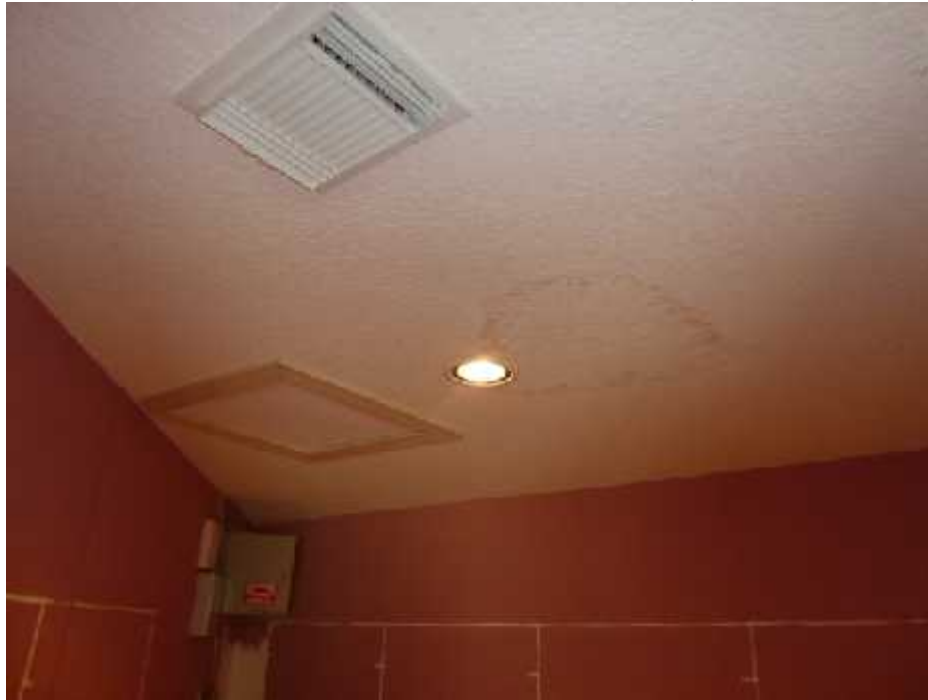
Ceiling in Master Closet
