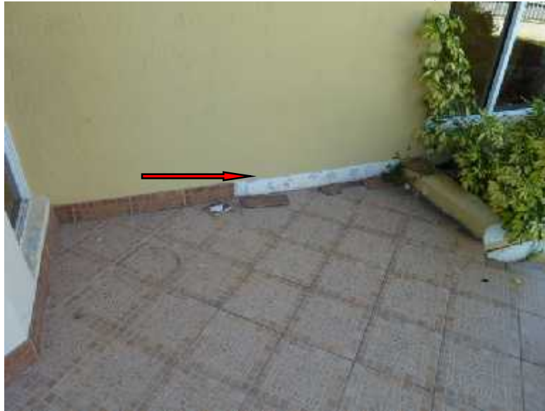
Photo: View of tiles on the Front Porch.
